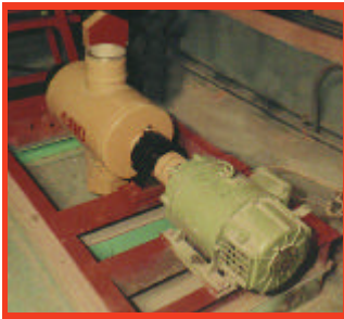
Radial centrifugal SHS installation
